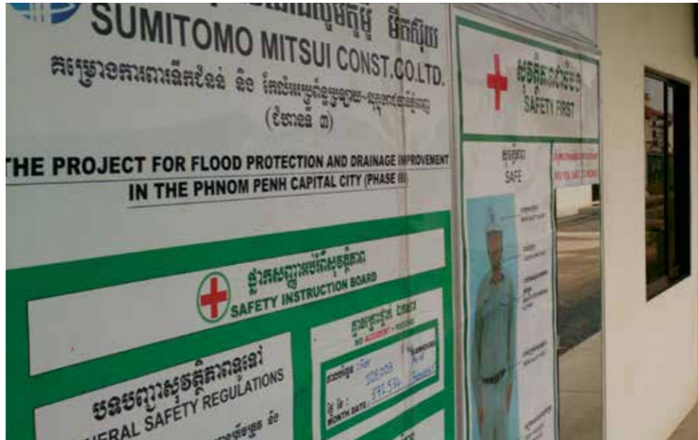
Japanese firms always prioritize safety principle at construction site
