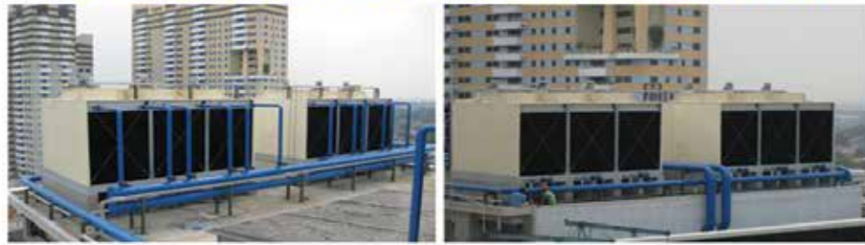
Cross Flow Square Type Model Cooling Tower from 100 ~ 10,000 tons
