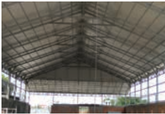
Roof Insulation on C Beams
