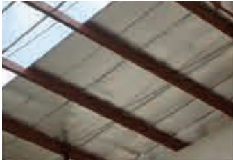
Roof Insulation on C Beams
