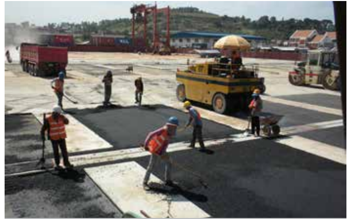
Asphalt Concrete for container terminal at Sihanoukville Port
