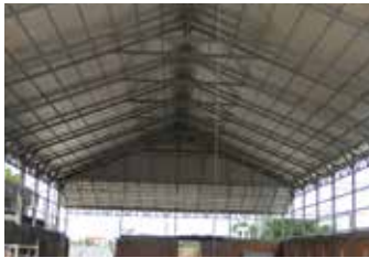
Roof Insulation on C Beams
