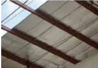
Roof Insulation on C Beams
