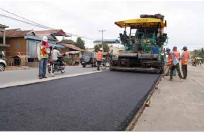
Asphalt road for National Road No. 1, Cambodia
