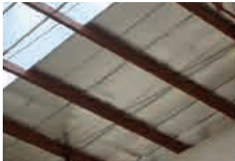
Roof Insulation on C Beams
