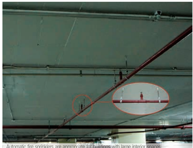
Automatic fire sprinklers are appropriate for buildings with large interior spaces
