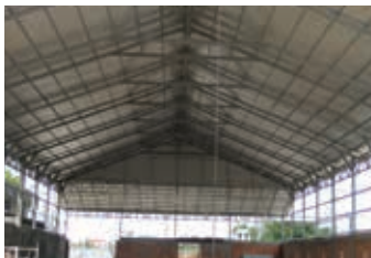
Roof Insulation on C Beams
