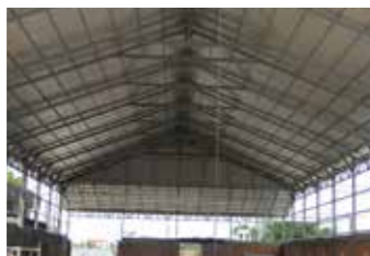
Roof Insulation on C Beams
