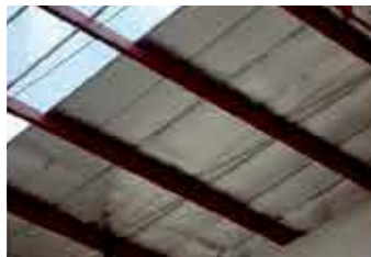
Roof Insulation on C Beams
