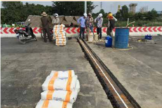
Concrete repair & protection systems
