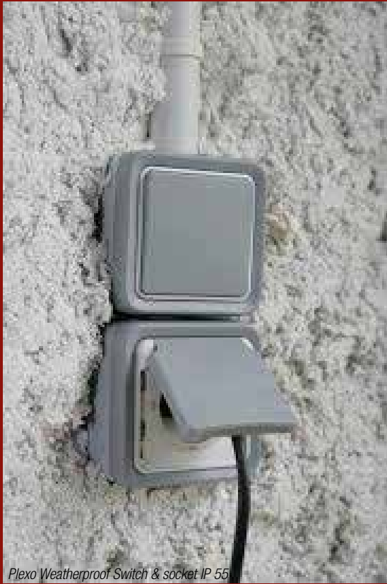
Plexo Weatherproof Switch & socket IP 55
