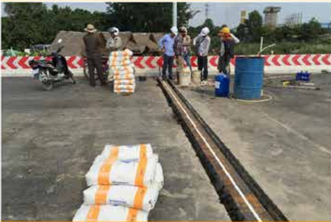
Concrete repair & protection systems
