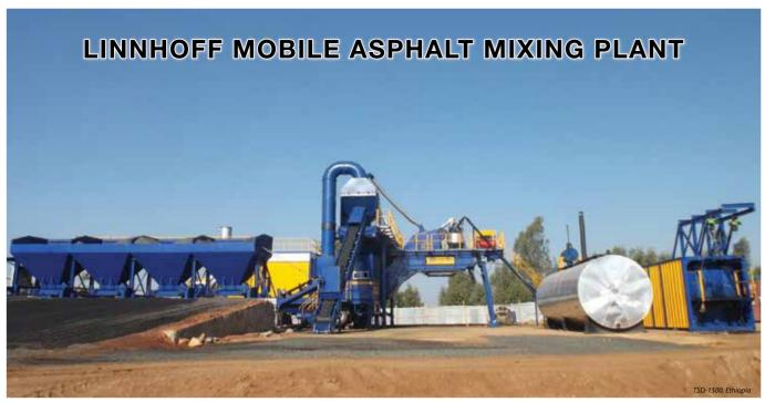
As a German manufacturer of asphalt mixing plants since the 1900s, Linnhoff has been committed to constantly innovate and develop more productive, efficient, and environmentfriendly asphalt mixing plants. Linnhoff Mobile Asphalt Mixing Plant series (TSD), with production capacities ranging from 60 tph to 120 tph, provides complete mobile solutions for quick dismantling and demobilization needs. To learn more about Linnhoff TSD asphalt mixing plants and their advantages, please contact us.
