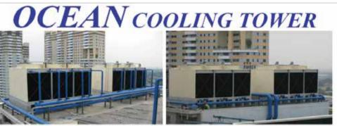
Cross Flow Square Type Model Cooling Tower from 100 ~ 10,000 tons
