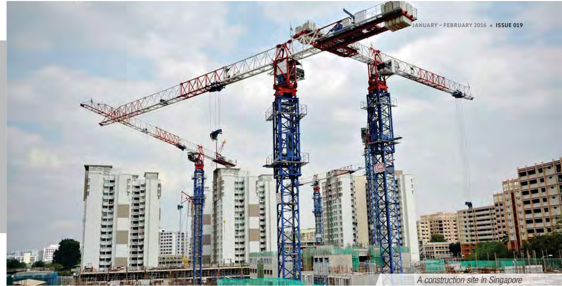
A construction site in Singapore
