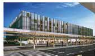
Tan Son Nhat Airport Car Park
