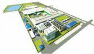
Heineken Factory Extension Cambodia
