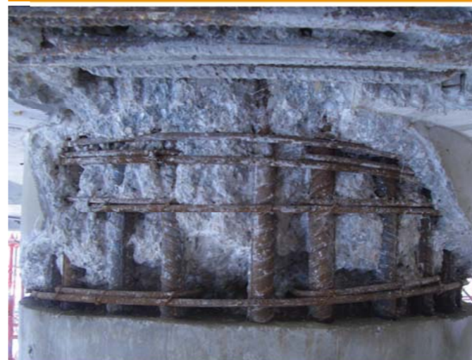
Concrete repair & protection systems
