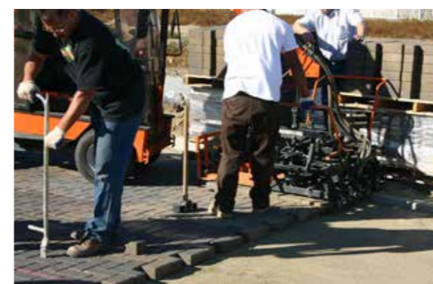
Edge Restraints of Precast Concrete Street in Sapporo City, Japan
