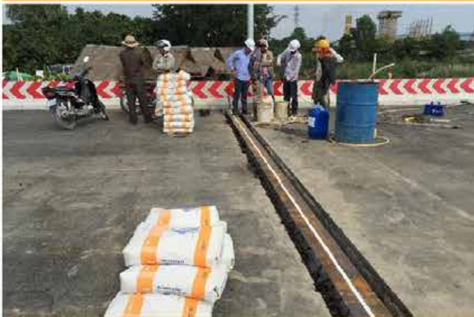
Concrete repair & protection systems
