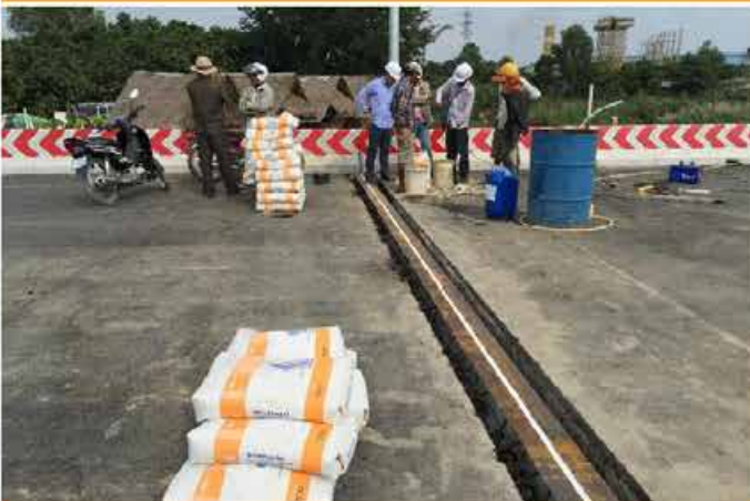
Concrete repair & protection systems
