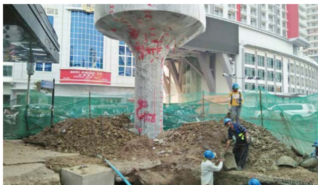
▼ Neang Kong Hing roundabout elevated walkway 50 percent complete
