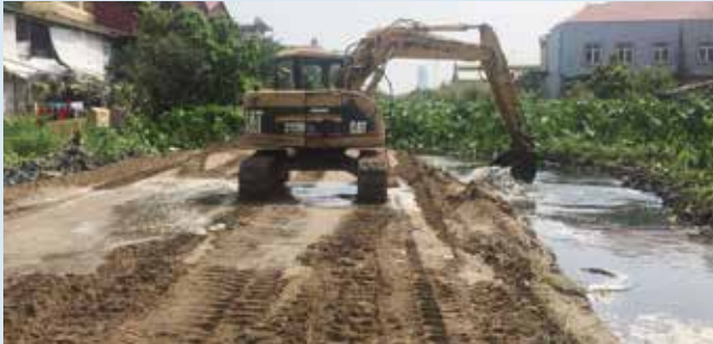
▼ Toul Kork water reservoir construction underway
