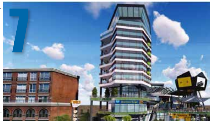
Downtown 93 Community Mall nearby Chbar Ampov bridge along Monivong Blvd (3,800sqm)
