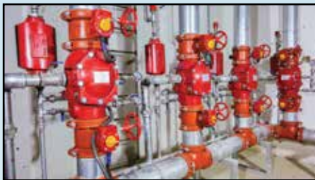
Commercial Building / Shopping Mall
