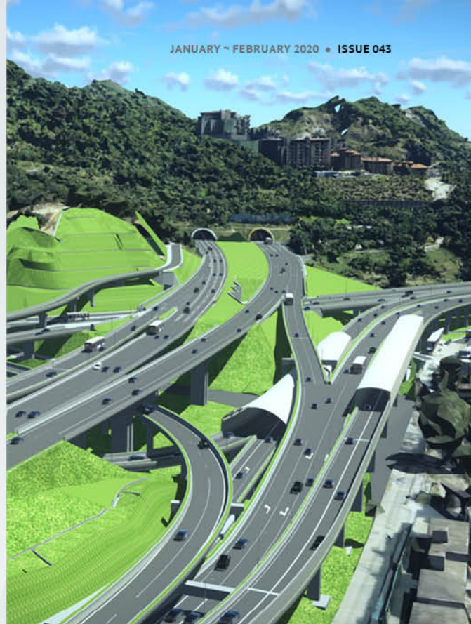
Innovative and Comprehensive Use of Digital Twins for Grade-Separated Junction Project in East Yan'gang Region
